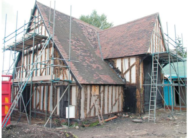
From survey digitals, LUH02, this view of the south west corner of the barn shows the lean-to extension, the projecting gable to the midstrey with brackets and the primary braced wall structure to the barn.
