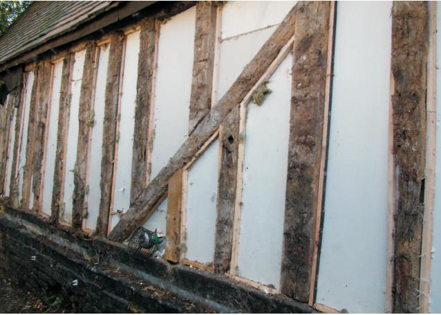
L23 shows the typical wall structure of the northerly aisle, set onto a good brick plinth the lower bricks of which are early but the top courses are later showing that a sill change has taken place.
