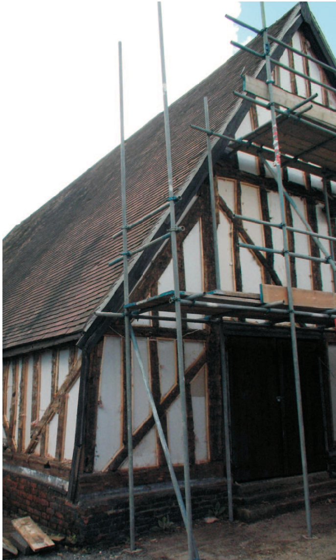
01 shows aisle end at west with the inner principle bracing the structure before the main rafters are fitted.
