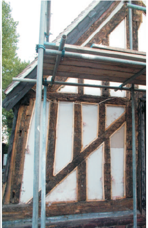
09 shows the truss design in more detail. The arcade post, aisle tie and aisle corner post are stiffened by the inner principle or shore. Structurally the lower primary brace for the infill should not be needed. But this is possibly a rebuilt end.
