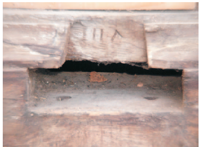
12 - reused timber in sill at western end of aisle is moulded and has mortises for meeting timbers. Suggest from a large window or panelled ceiling.
