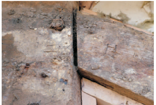
17 - marks where wall brace meets upper part of stud on aisle wall.
