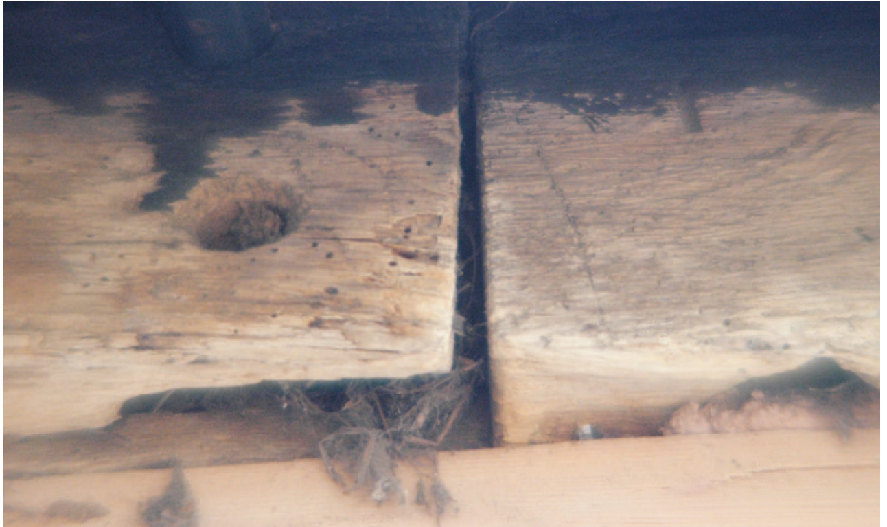
13 is scarf number I from the west in the aisle walling. Face halved and bladed type. Chiselled I.
