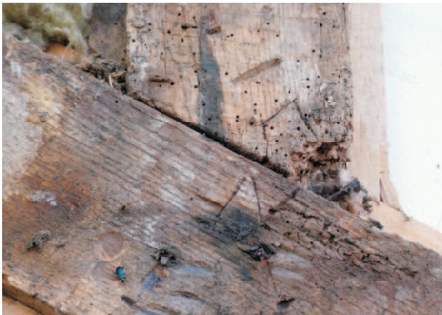
16 - Carpenters assembly marks chiselled as are all to the construction. This where stud meets brace.
