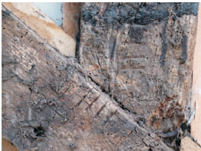
15 - more examples of assembly marks IIII where stud meets brace.
