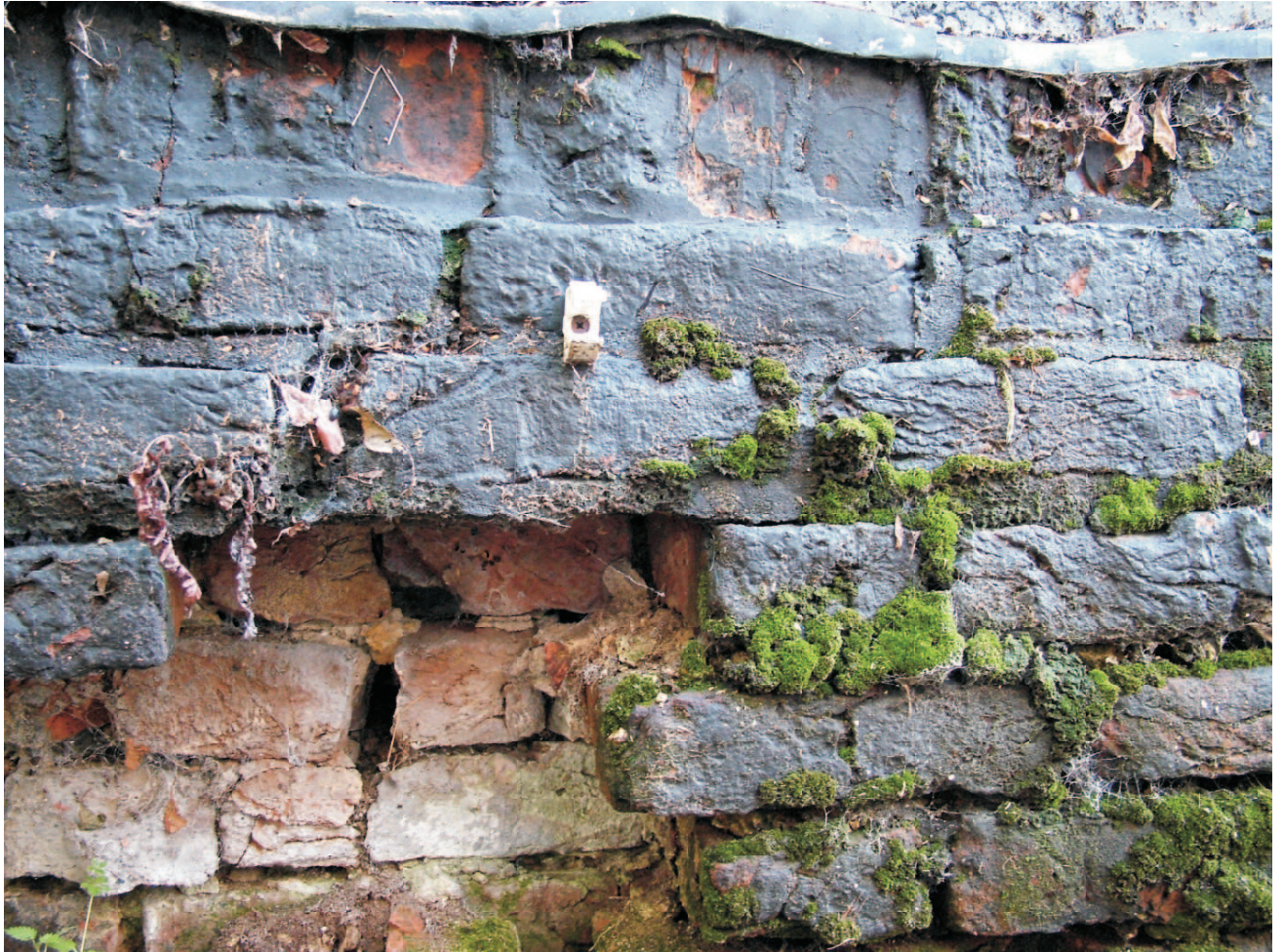
33 shows the plinth towards the northern end with early brick and later on edge brick under sill.
