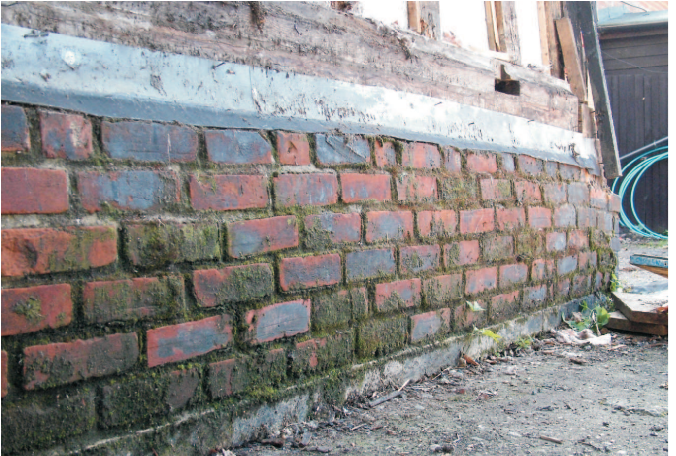
37 shows the plinth towards the western end where the barn has been reduced and this is C19 brickwork.
