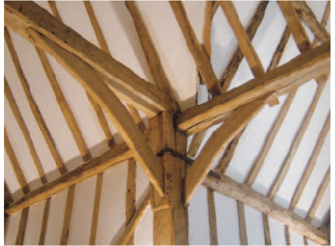
Owners digital 48 - to E showing storey post to midstrey with added iron tie to midstrey wallplate.
