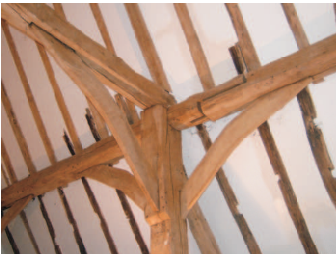
Owners digital 17 - to W showing top of arcade post, cranked arch braces and the edge halved and bridled scarfs to the plate. Note the reuse of crown post roof rafters in the construction that have most likely come from an earlier domestic building as they show signs of sooting from an open fire.
