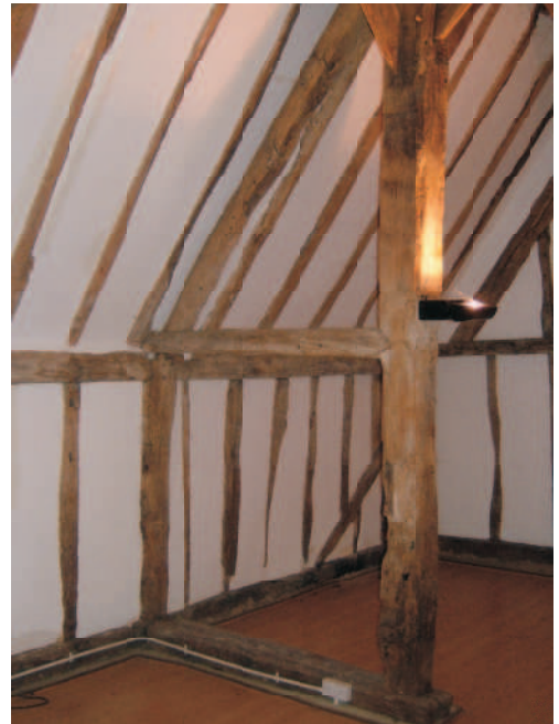
Owners digital 27 - to NE showing the lower part of third arcade post with sill return to aisle.
