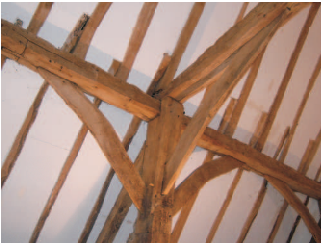
Owners digital 25 - to N showing third arcade post to aisle side and edge halved and bridled scarfs to the arcade plate.
