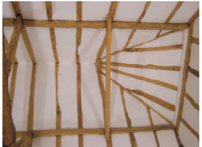
Owners digital 76 - to NE showing the roof end construction with half hip. The hip rafters rise to a very high set saddle not leaving space for gablet ventilation.
