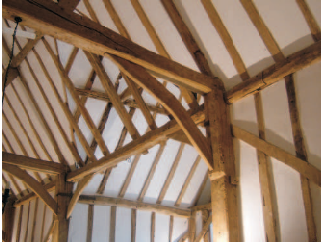
Owners digital 66 - to E showing the entry into the midstrey with storey posts and the slightly cranked arch braces to the tiebeams. note the scarf in the wallplate is a face halved and bladed as appears in the aisle wallplate.
