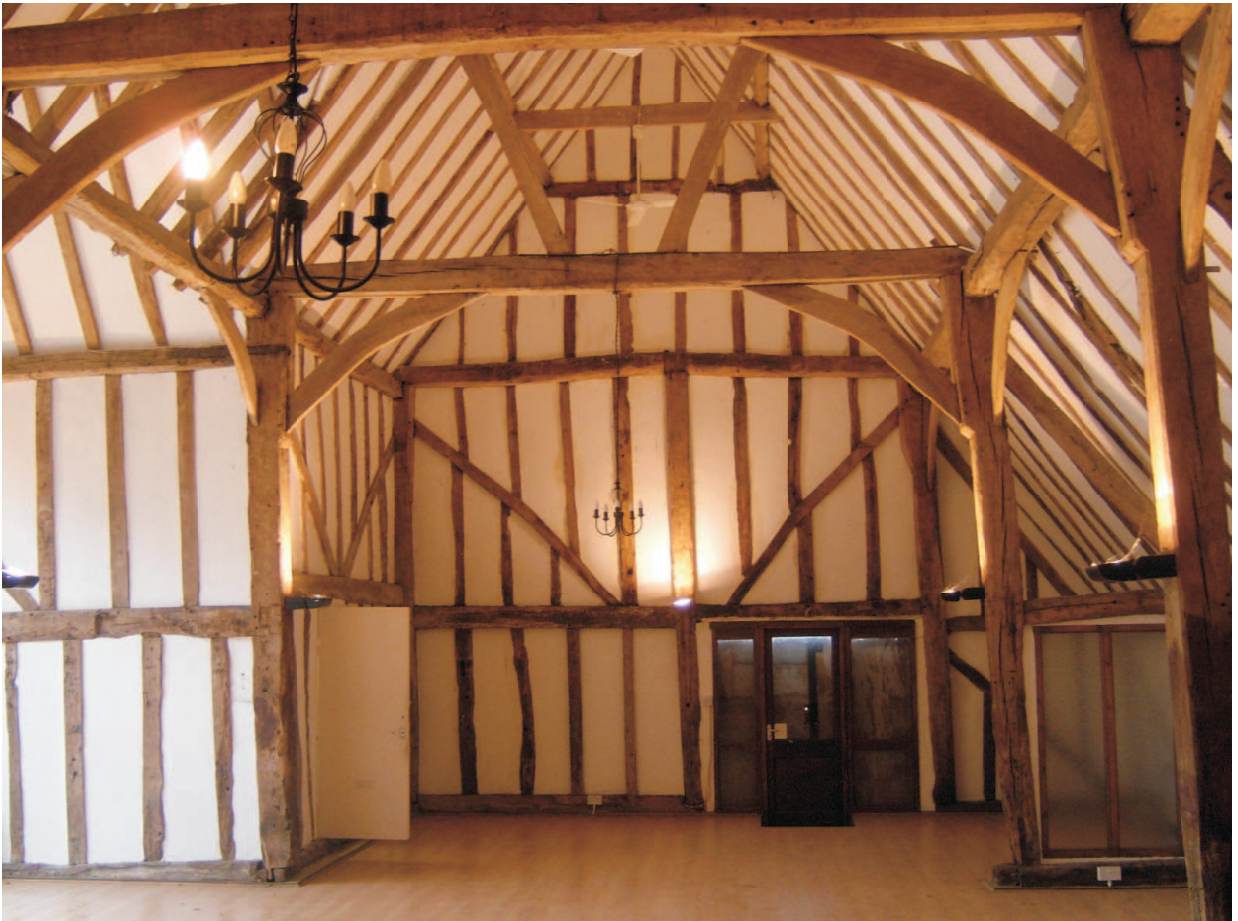
Owners digital 99 - to SW showing the bay beyond midstrey with arcade posts and aisle. This possibly reduced by one bay as infill to aisle the posts and the gable end are changed detail.
