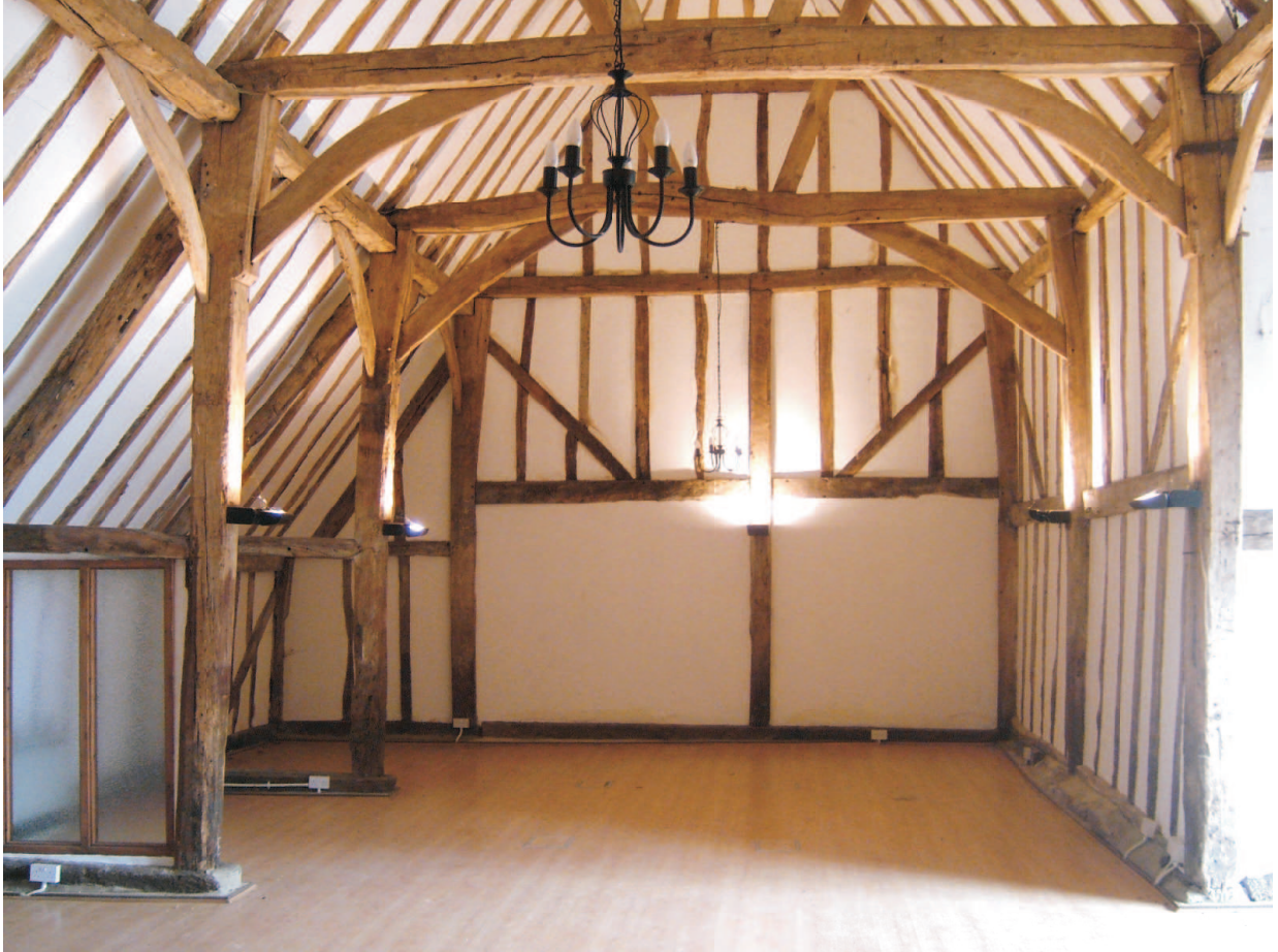
Owners digital 94 - to NE showing two bays beyond midstrey with arcade posts and aisle and the more original end of the barn.
