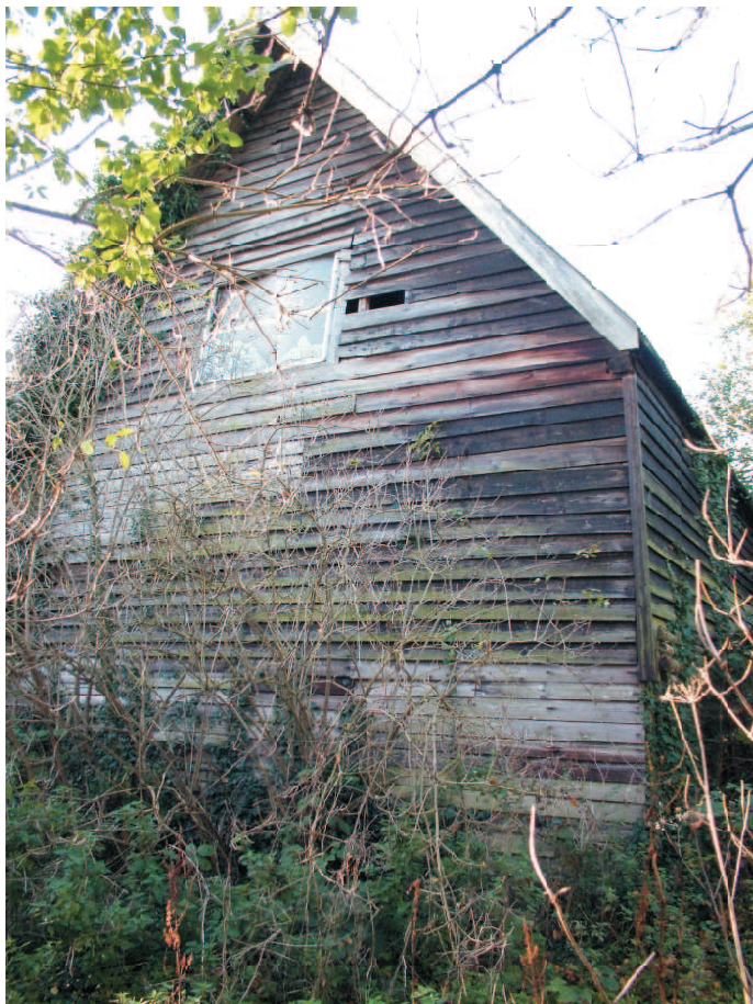
View from the north east showing one of the inserted windows and a mix of modern weatherboard cladding.
