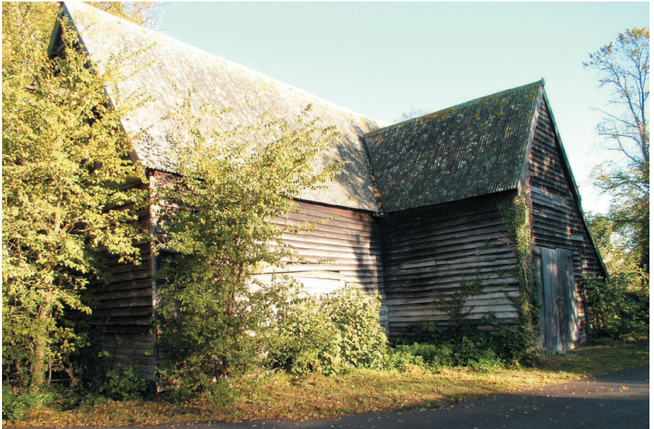
Outside view of the barn from the south west. High pitched roof and original midstrey. Main doors of porch reduced in height and width. Later lean-to to the east side of porch.
