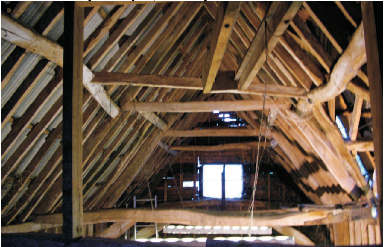
View at tiebeam level looking east. Joggled framed side purlin roof collars mortised into principle rafters and birds mouth intermediate collar above the midstrey bay. End of Crittall installed trackway at top of photograph.
