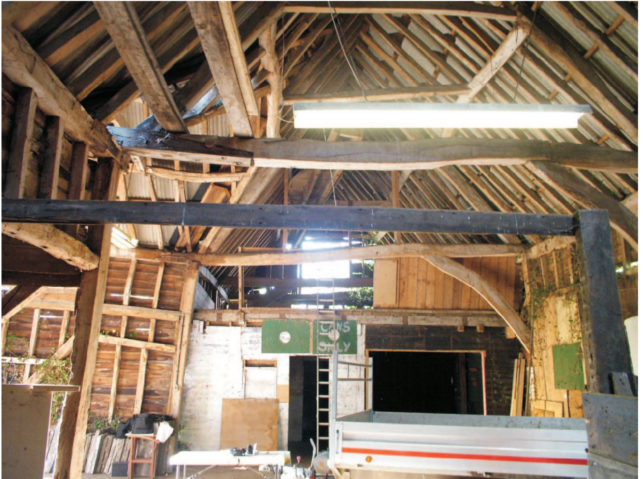
General view looking west to inserted floor beyond the midstrey opening. Under the floor divided into two rooms with no natural light. Note large serpentine bracing to rear wall.
