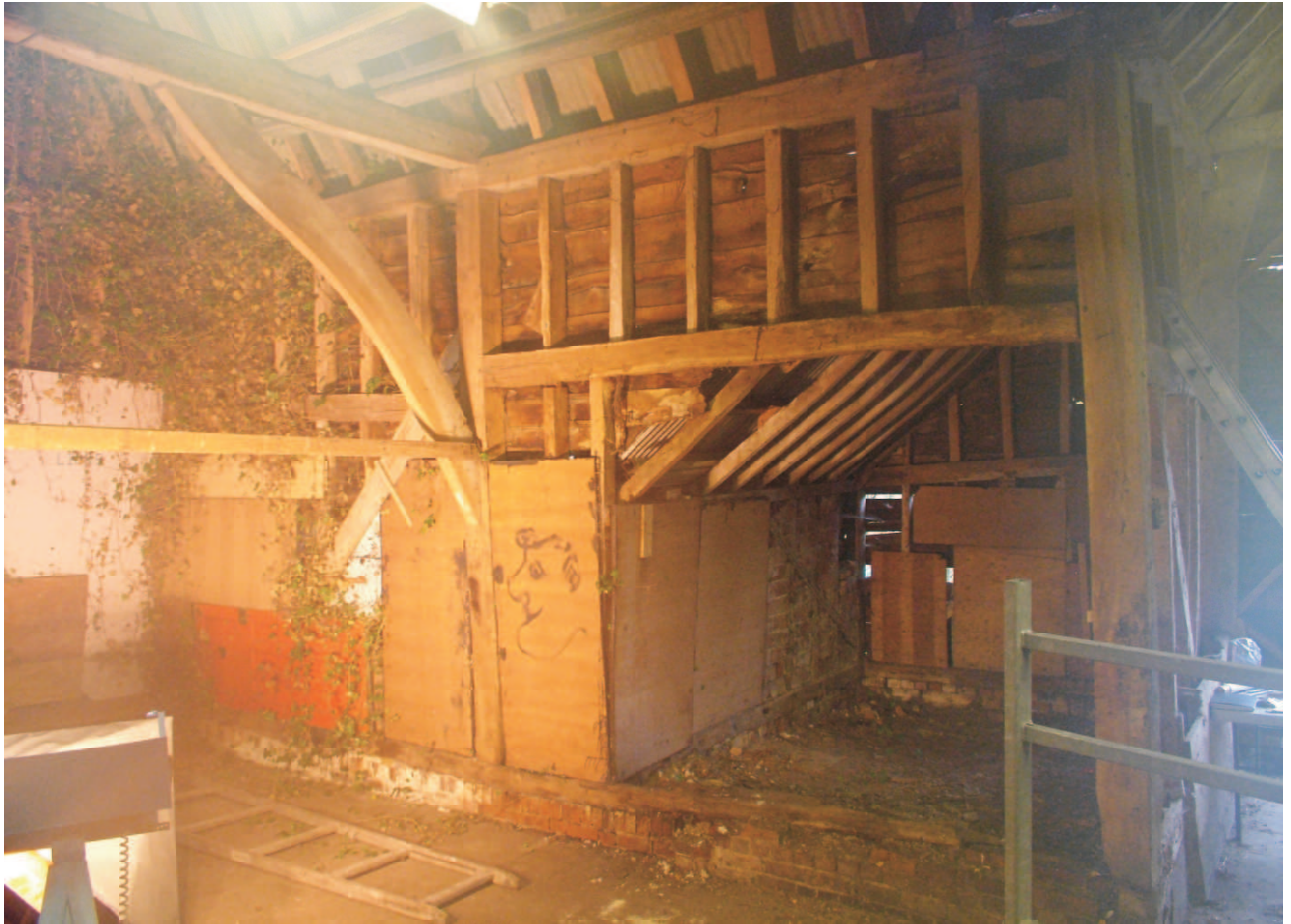
View towards the south east into the lean-to. Note heavy main framing timber to barn and large serpentine brace. Visible brick plinth of barn with top course of brick on edge as is remaining wall infill to lean-to.
