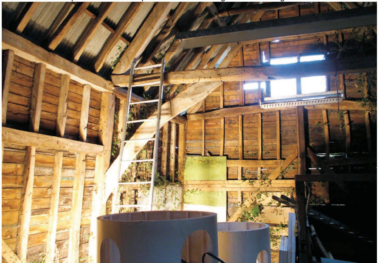
View towards the north east clearly showing the unusual framing to the barn. High heavy section primary wall braces with a midrail into them two-thirds of way from sill to wallplate. Stud lengths vary as to position in barn, being unusually short above midrails in bays with primary braces..
