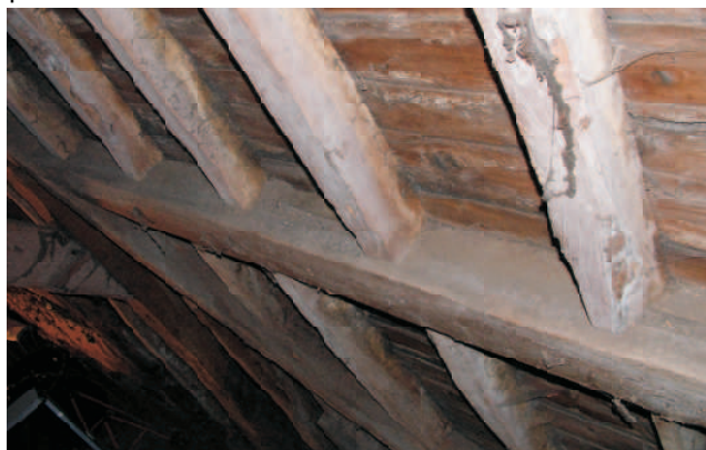
Most examples in the barn have the long mortise as the lower element. They have filled over the years and are not easily visible within the structure unless viewed from a high level.
