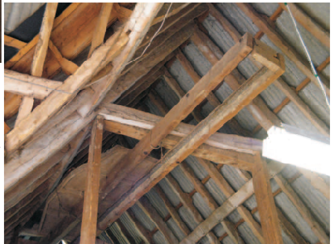
Run of intermediate lower rafters in the fourth bay from the east. Note the four from the left made from one tree sawn through to produce four good rafters. As long as the saw cuts or conversion follows the natural grown shape of the tree all pieces will have maximum strength for section size. Other examples of this method of conversion occur within the barn structure.
