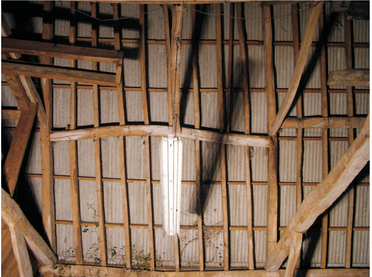
Roof of the main barn. Joggled side purlin providing strong single joints into the principle rafters above and below collar mortise. The lower run of intermediate rafters are mortised and pegged at the upper end into the purlins. The upper run of rafters not pegged. Intermediate birds mouth collar in most bays.
