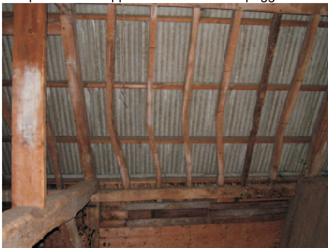
Roof of the main barn. Joggled side purlin providing strong single joints into the principle rafters above and below collar mortise. The lower run of intermediate rafters are mortised and pegged at the upper end into the purlins. The upper run of rafters not pegged. Intermediate birds mouth collar in most bays.
