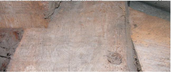
Example of face mark to one of the tiebeams. This shows the fair face produced from hewing the timber and is used as the set-out face when marking out the frame. Were visible on some tiebeams and principle rafters.
