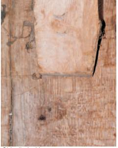
Chiselled with gouge carpenters assy. marks to arch braces and storey posts.
