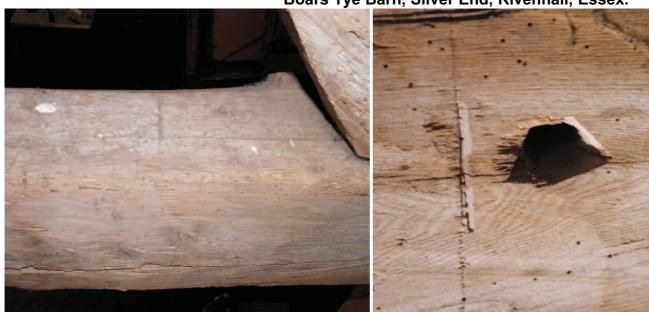
Scribed and chiselled marking on tiebeams. For alignment and setting out of frame, to right is detail of how the chisel was used to accentuate the scribed horizontal and vertical lines. Hole shows start for non-pointed auger.
