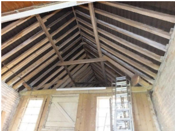
Inside showing the side purlin roof and later partition board panelling, doors and windows.
