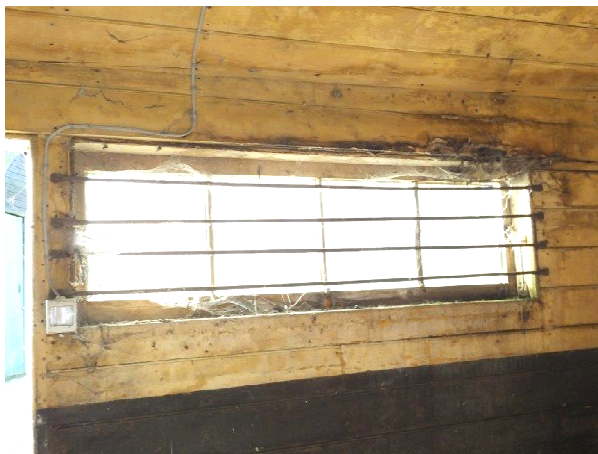
Top hung four light windows with inner security bars and hook and eye opening stay.
