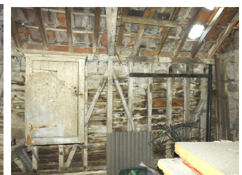
Rear wall of tack room primary braced.
