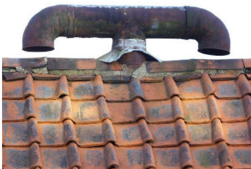
Roof vent and single Roman profile clay tiles.
