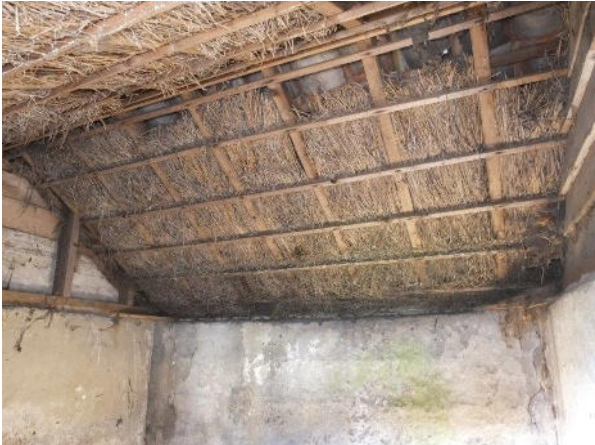
View inside showing straw insulation.
