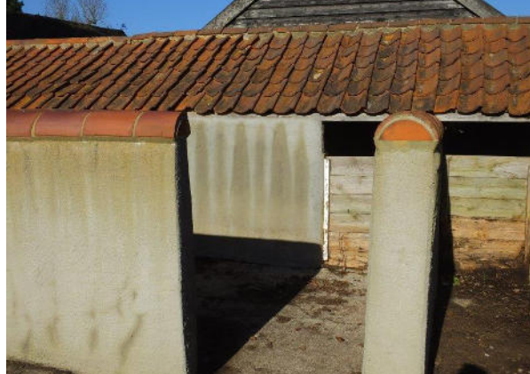
View into one unit. Boarded entry. Pantile roof.
