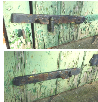
Safety drop over latch at bottom of lower door shown closed & open.
