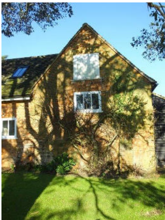
South gable with filled loading hatch. Original carriage shed brickwork with diagonal pressure marks and later lean-to with horizontal pressure marks showing 18 th & 19 th century work.
