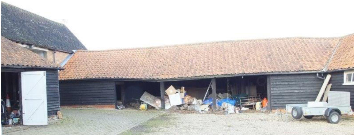
Cart lodge range with boarded front to two outer bays. Roofed in single Roman profile clay tiles.
