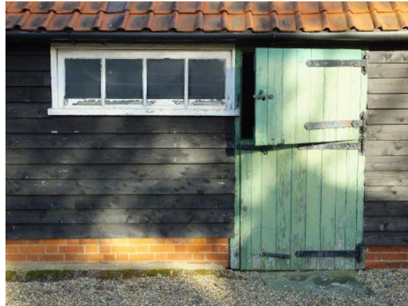
Stable doors and top hung window detail.
