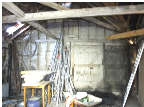
Tack room division wall to first stable.
