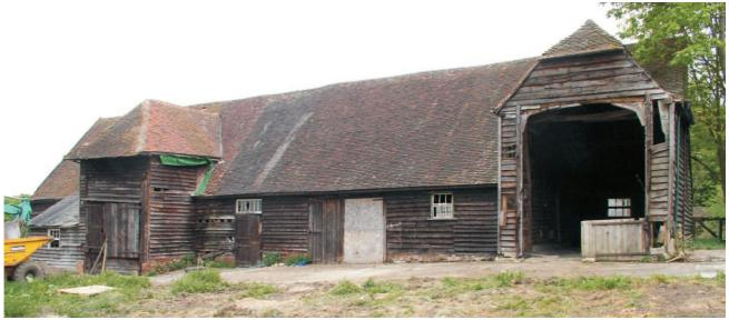
The barn in 2007. Note the doors to the north midstrey have been reduced in height. The northern stable door is similar but with a glass light above. The other door has changed completely and a window has been added between it and the south midstrey, now devoid of doors.
