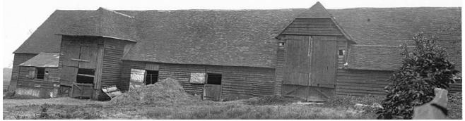
Extract from 1920 RC photograph showing barn with the two bays now removed at the south. A lean-to also existed for at least one of the bays. Also note that stable doors had already been inserted into the bays of the barn to the north of the older section of the barn.
