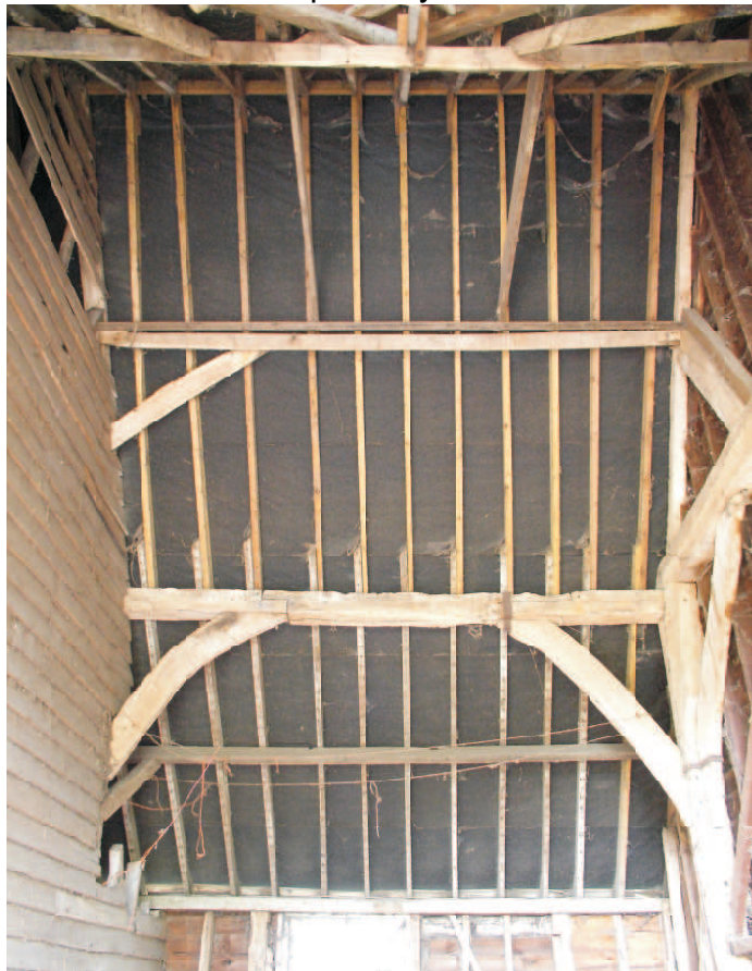
(290) West wall (rebuilt) and roof bay 1-2
