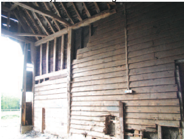
(293) North side porch wall with elm boards
