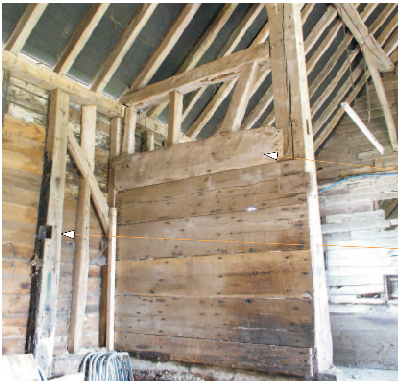
(256) Elm board infill to aisle wall. Top board was outer board of tree and axe converted before through sawing the other boards.
