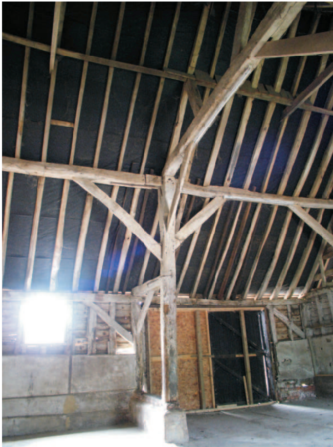
(241) View to post 3D the intermediate of the seventeenth century rebuild. note the face halved bladed scarf to the arcade plate.
