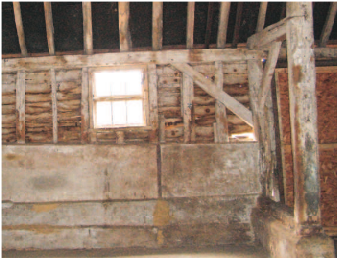
(146) Aisle arch bracing to the bays of the seventeenth century rebuild.
