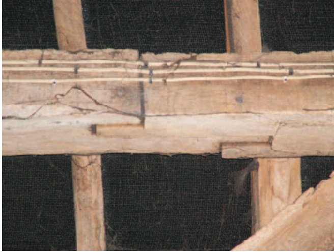
(143) Typical face halved scarf to arcade plates other than in bay 1-2.
