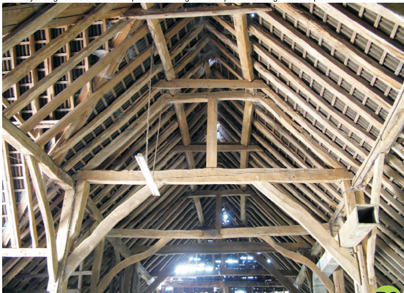
Photo 208. Inside view above aisle level looking to the south east with heavy duty trunking on arch braces, crown strut from tiebeam to collar with extra part truss with serpentine bracing at mid bay.
