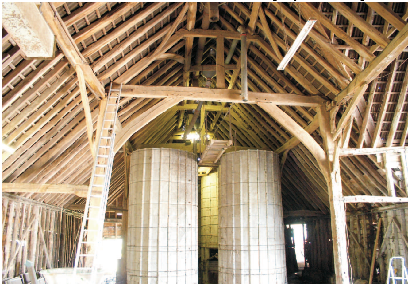
Photo 172. Inside view looking to the north west with concrete grain silos & associated operating gear and walkways. Original aisle tie to left replacement to right. Brace problems to right arcade plate.
