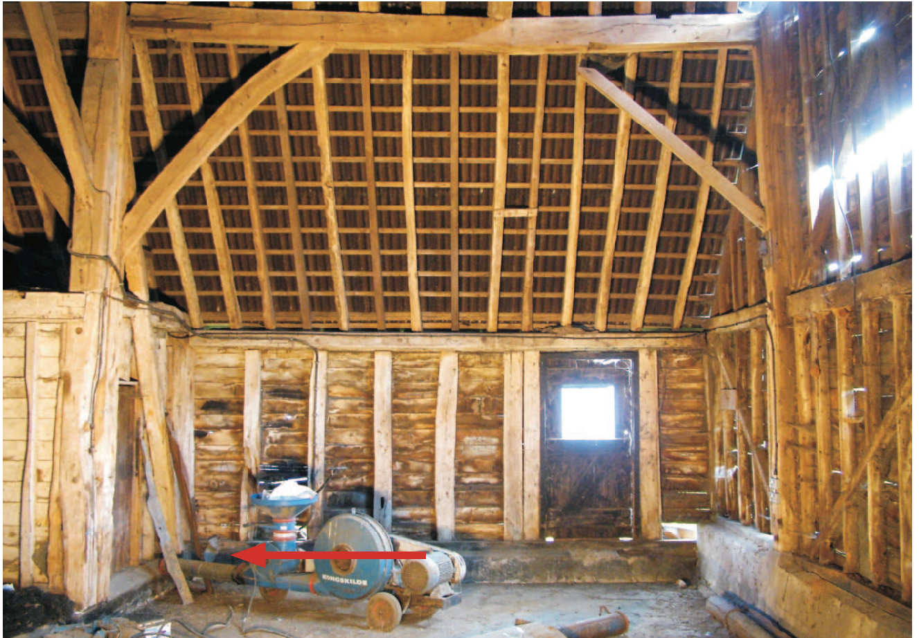
Photo 76. One of two bays with original walling. Wall D, Bay 1 - 3. Good relatively large section timber typical of middle sixteenth century. Later door inserted in nineteenth century. Aisle roof rebuilt as is end wall.
