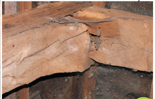
Photo 48. Typical ridge joint to main trusses showing swelled end of reduced principal rafters.
