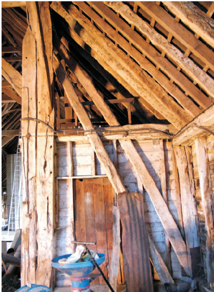
Photo 78. View in direction of arrow above showing aisle tie and shore with extra shore but brace to return sill missing.
