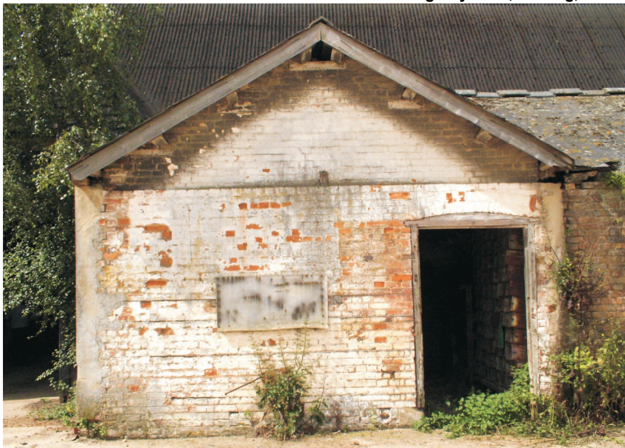
Photo 5. View on 6 - 6A wall F. Broken brick to outer edges shows this was internal wall. Original doorway.
