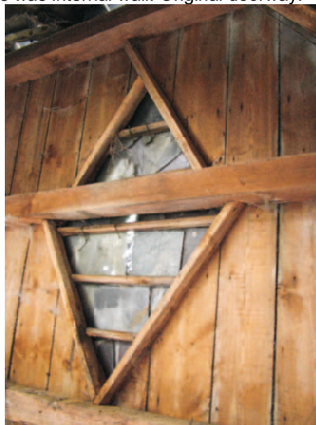
Photo 133. Detail of roof light.
