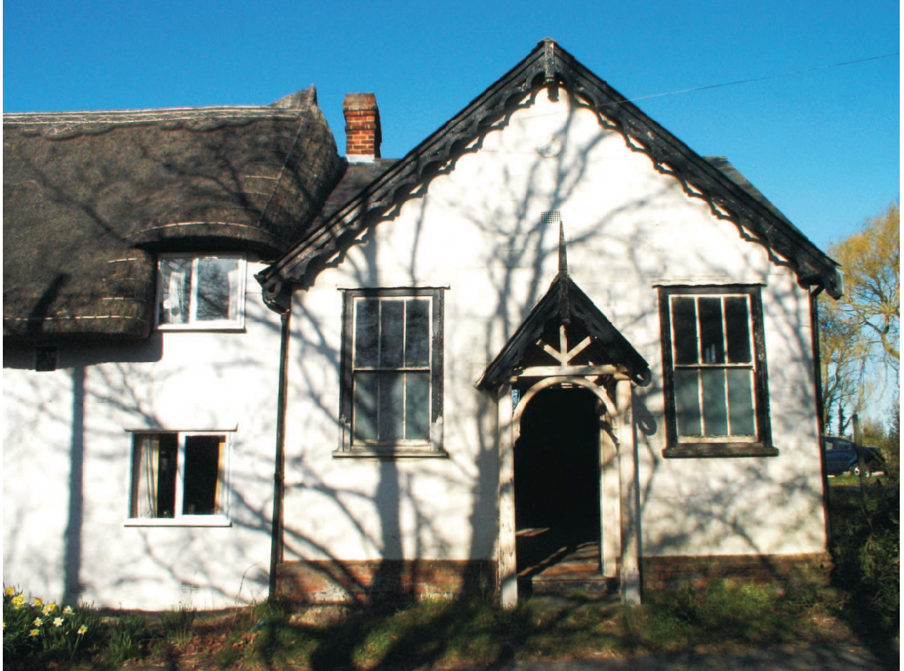
View from the east with timber porch to entry door and two sash windows. Main and porch gables have decorated and pierced bargeboards. Roof is slate and the plinth is Flemish bond brickwork. The lime plaster render is ashlar marked. The cottage is attached.
