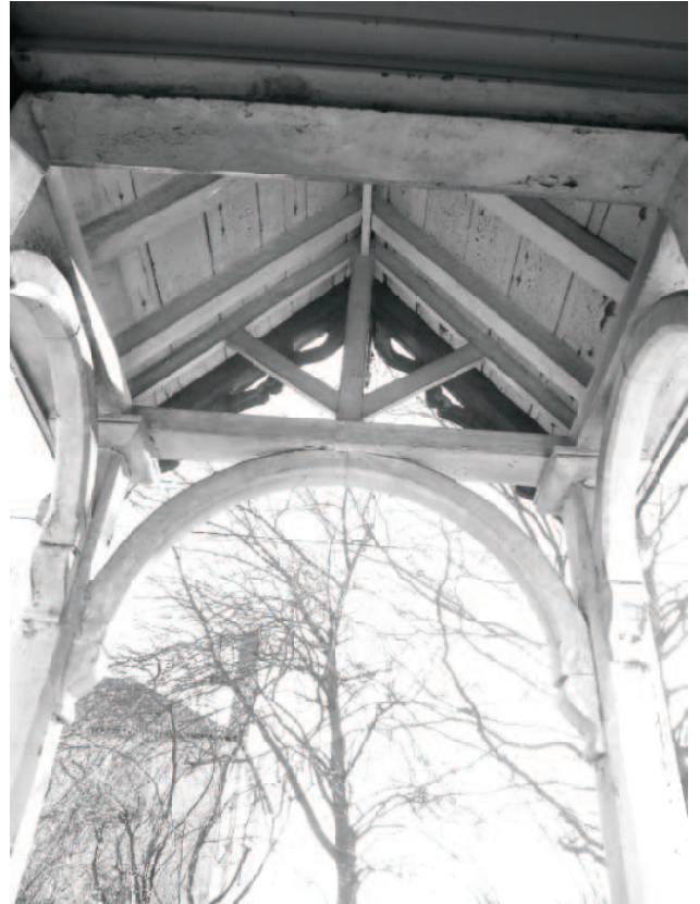
Inside view of porch showing king post supporting the ridge board and rafters down to plate.
