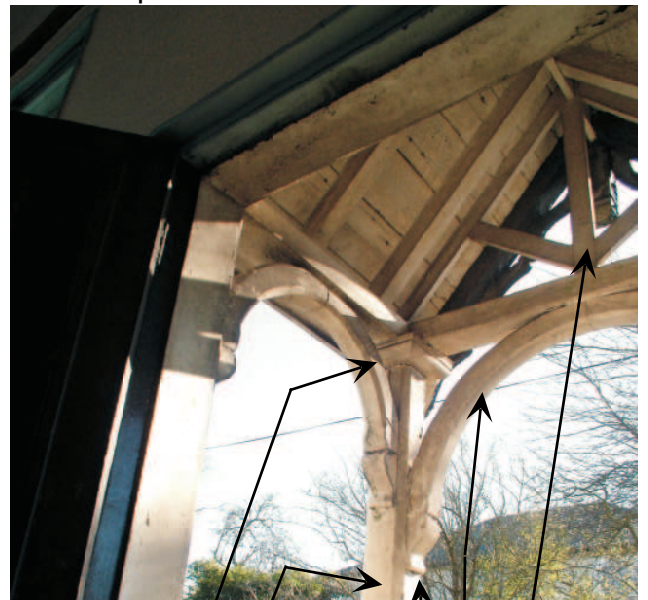
Inside view of porch showing king post supporting the ridge board and rafters down to plate.
