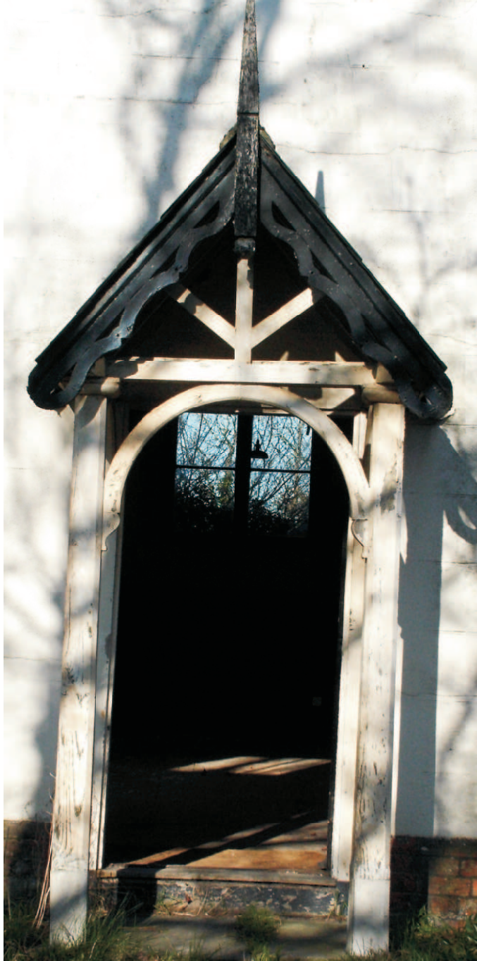
Front of porch with central finial.
