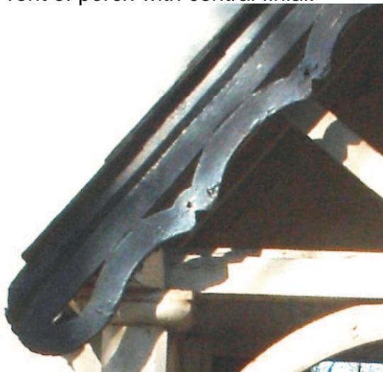
Detail of bargeboard.
