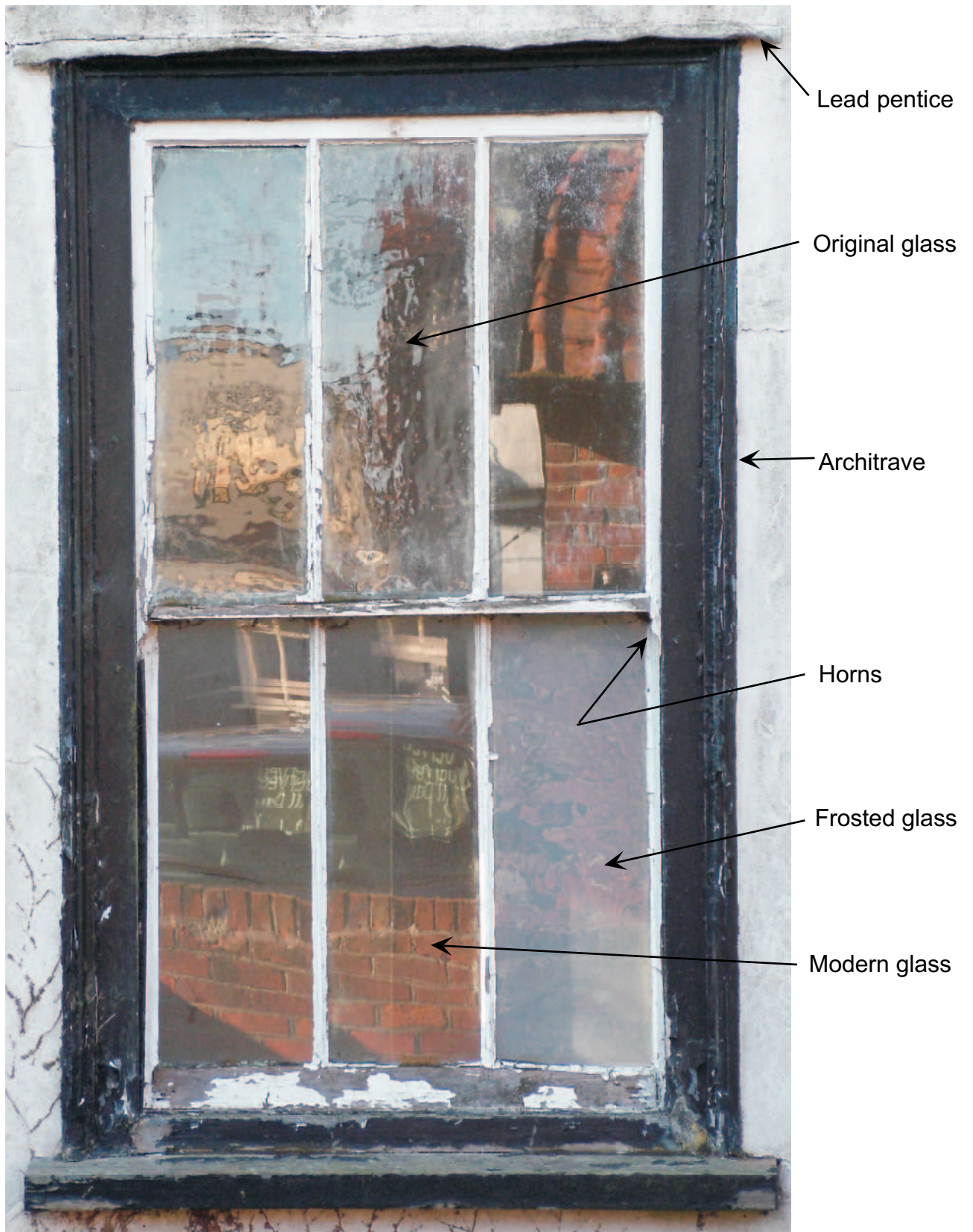
Typical sash window details.
