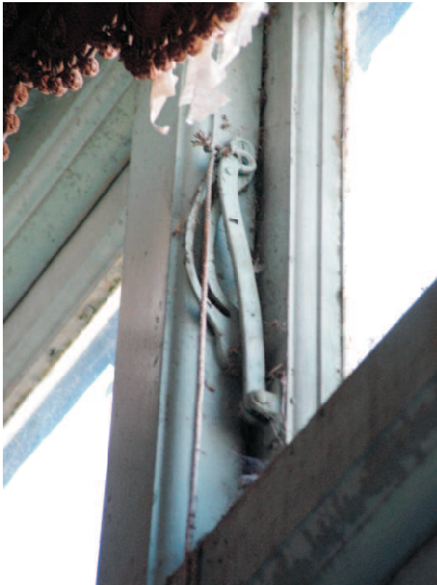
Mechanism on large west window to open pivoting lights with pull rope.
