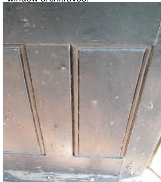
Detail of lower front panels.
