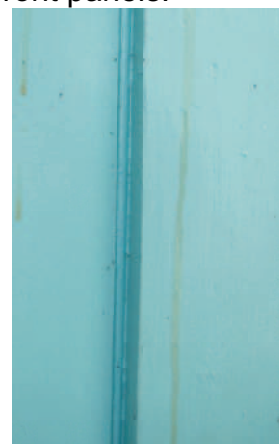
Cockbead edge to inner panelling.
