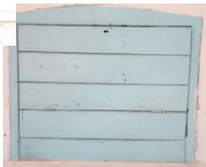
Fireplace opening shown with timber flap both open and closed
