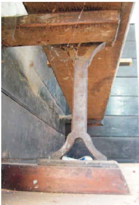
Fixed bench at east end with cast iron support
