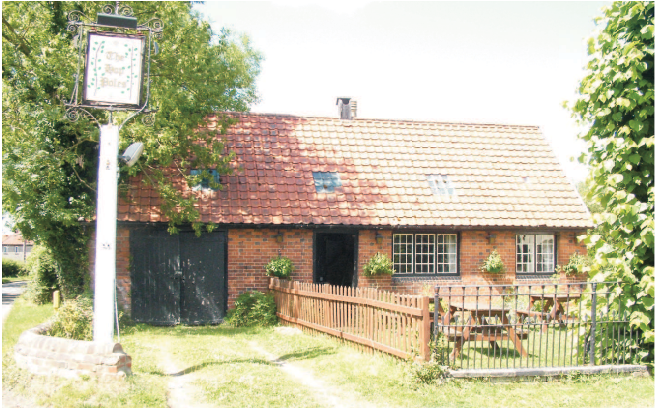
Front view of the forge building with boundary wall lowered and partially removed.
