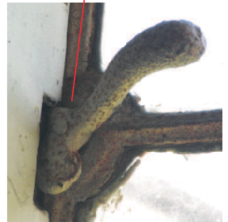
Lever handle - cast iron
