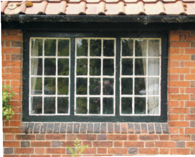
Fixed window, timber frame with CI casements
