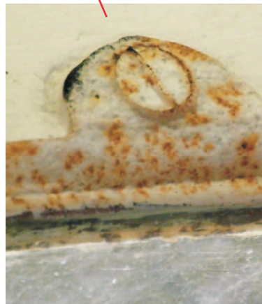
Fixing boss on all windows top & bottom of each
