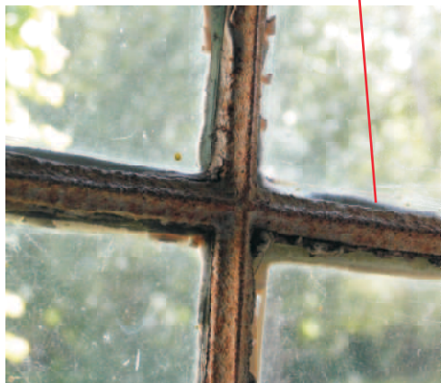
Section of cast iron casements
