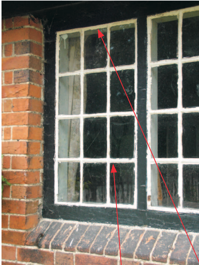
Cant sill bricks to openings
