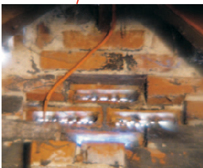
Air bricks at top of east gable
