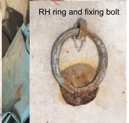
View towards rear wall with board mounted tying rings and the heads of board fixing bolts.
