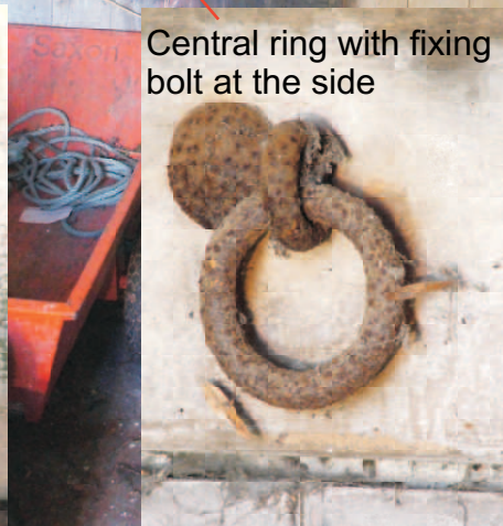
View towards rear wall with board mounted tying rings and the heads of board fixing bolts.
