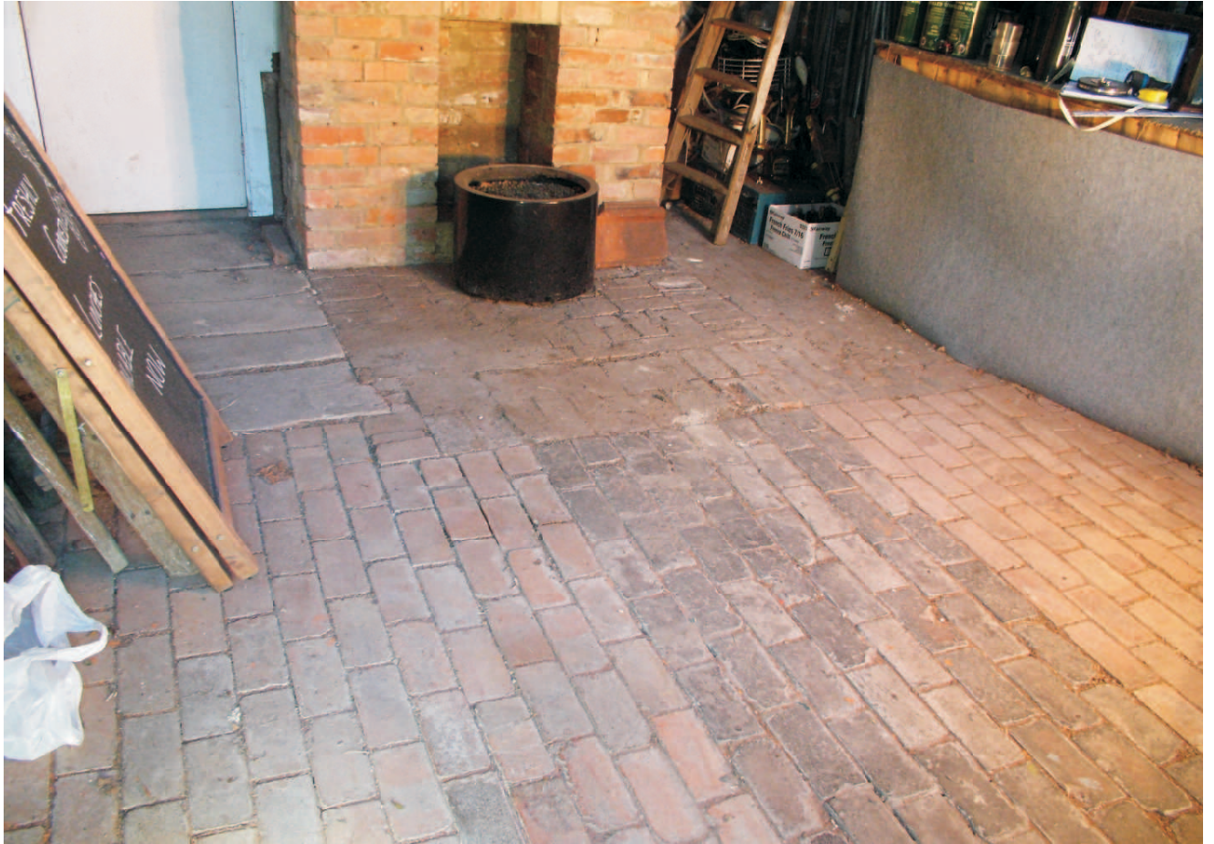
Central area showing the various brick finishes to the floor hearth area and boarded area
