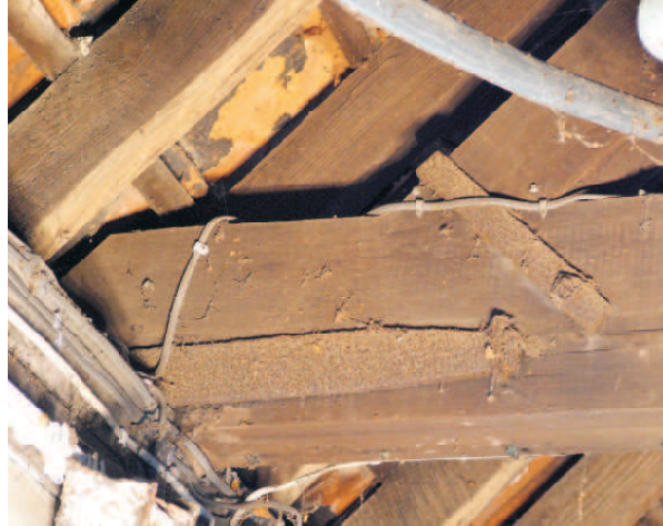
Tiebeam & principal rafter iron ties
