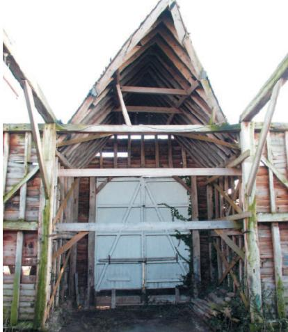
A general view looking north through the nave of the barn, A, showing the rear aisle main trusses to tiebeam level and salvaged timbers from the collapsed roof. Stabilising timbers are bolted through the structure and into the midstreys.
