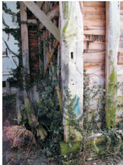
Barn A. Mousetead mortise in post at midstrey to allow threshing division.
