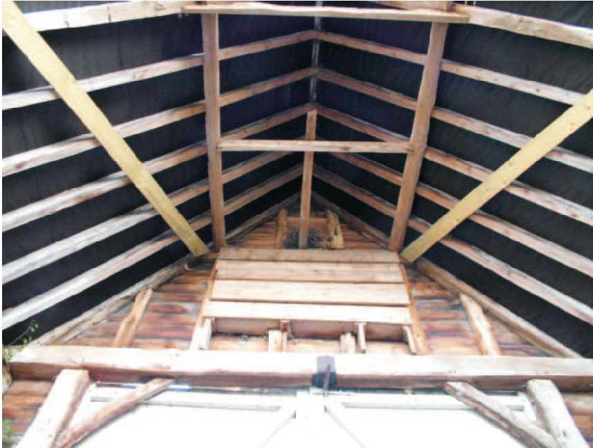
Barn A. View up to gable of southern midstrey showing pigeon box that appears to be a nineteenth century insertion.
