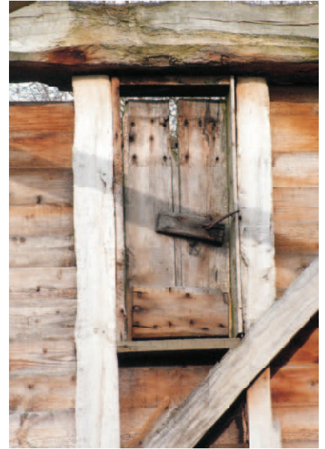
Barn A. Small inserted door high in the north gable wall, use unknown.
