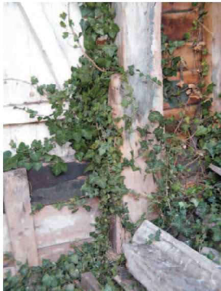
Barn A. Example of leap board slots at base of midstrey door post.
