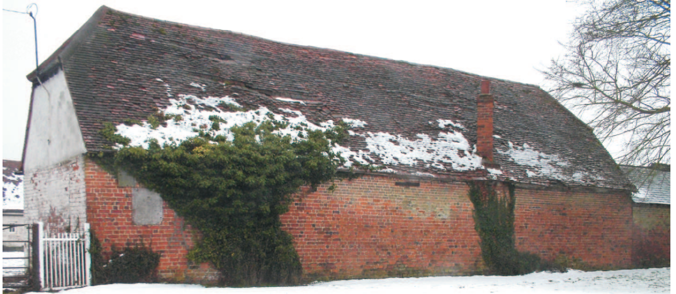
Building B. Main eighteenth century block from the north. Originally a window behind creeper.
