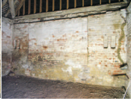
East wall with infilled doorway and brick formed vents.
