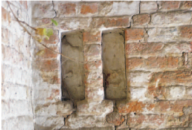
Detail of a brick vent window in east wall.
