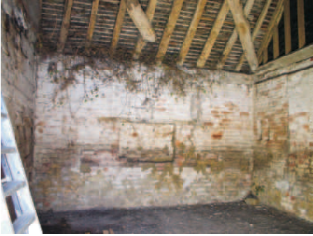
Building B. Carriage shed, north wall with infilled window.
