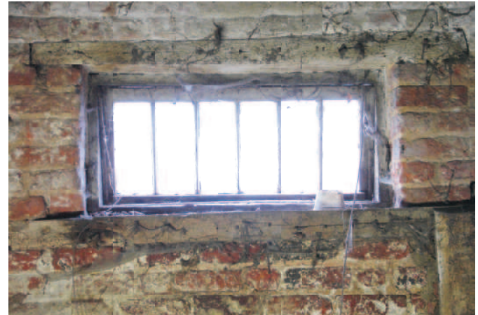
Detail of pivoting timber window in south wall.
