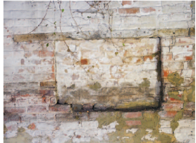
Detail of infilled window in north wall.
