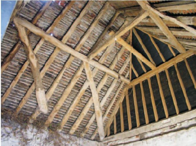
Side purlin roof, Carriage shed, modern rebuild hip end.
