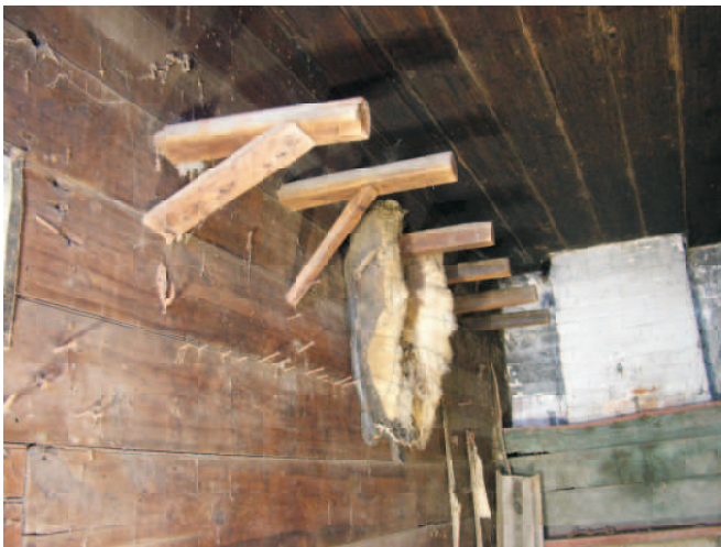
The left side has heavy timber brackets for collars and heavier harness items.
