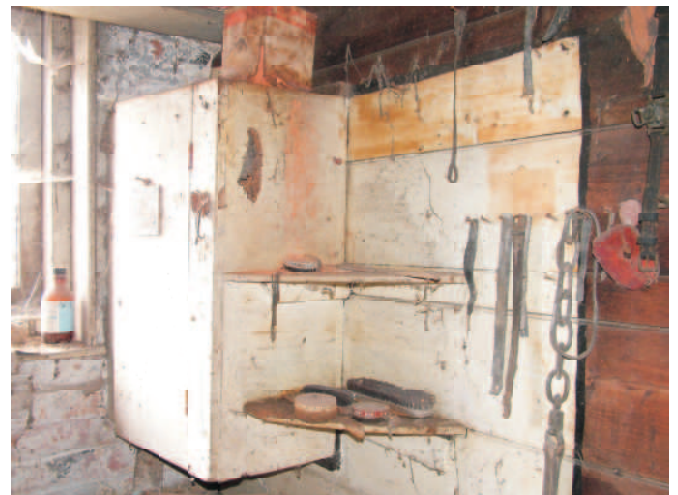
Above the bench is a secure store cupboard on a board backing with corner shelves.
