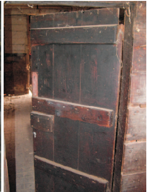
The good eighteenth century entry door from the Nag stable has a key lock.
