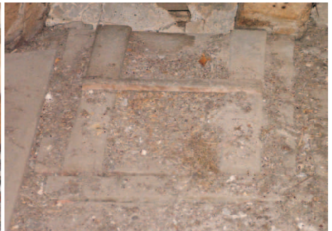
Cover to hay drop hatch (1 of 3) to hay racks below.
