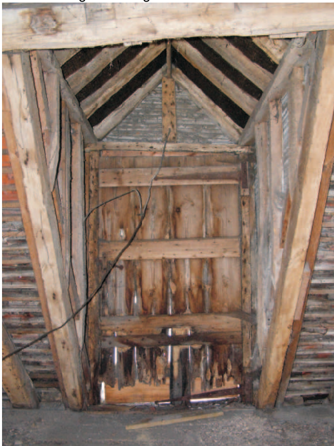
Gabled roofed timber framed dormered loading door to the farmyard. Good wide boarded unbraced door suggests eighteenth century as do the long fine hinges.
