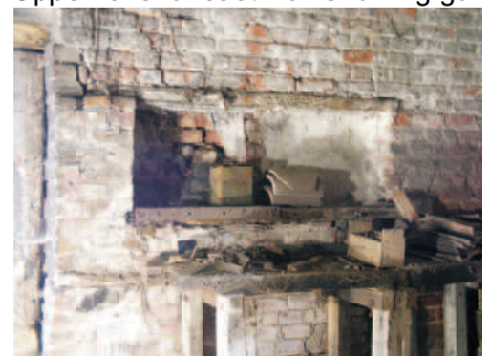
Plastered niche in front wall.
