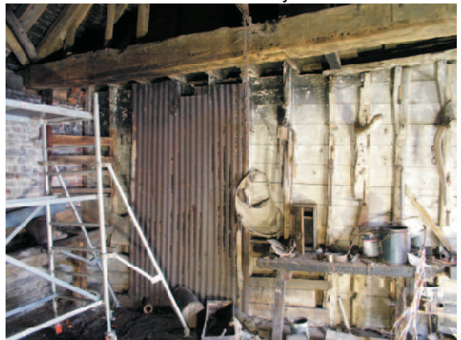
Lower section of east wall showing timber structure.
