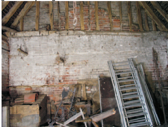
End wall with similar brickwork to main walls. Remains of vertical boarding survive with lacing pieces in wall.
