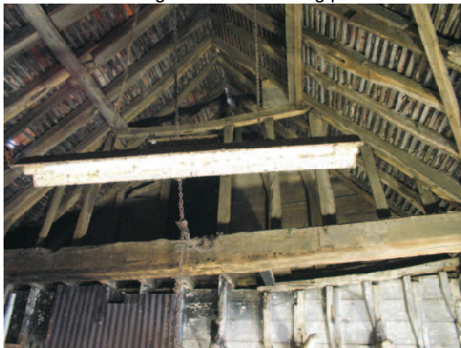
Upper level of east wall showing gallery to hay loft.
