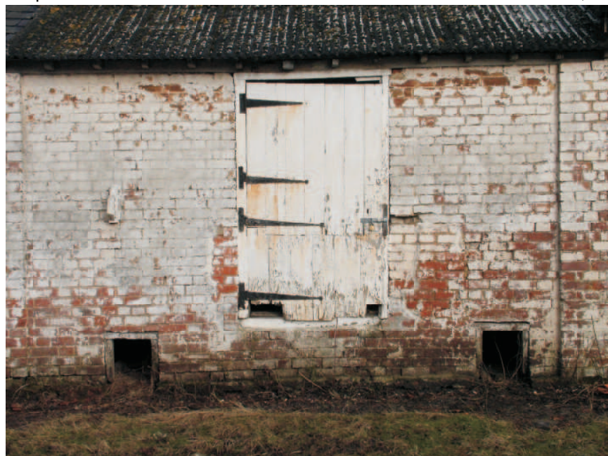
Front of granary build with raised floor and dog kennels under.
