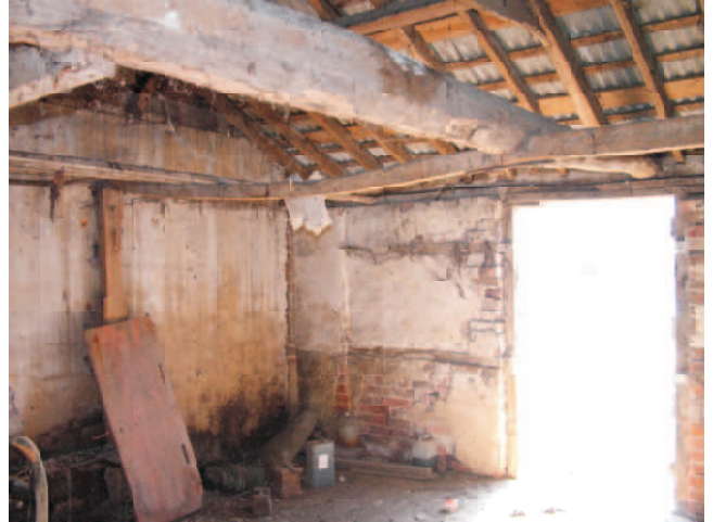
View to front wall showing plastered finish most likely boarded below lacing pieces.
