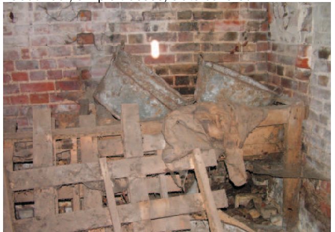
Feed trough & marks for hay rack on wall.
