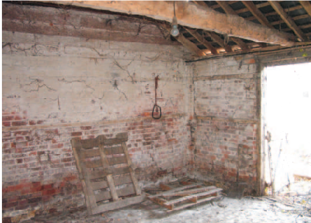
Building B west. Central Loose Box - to south/east.
