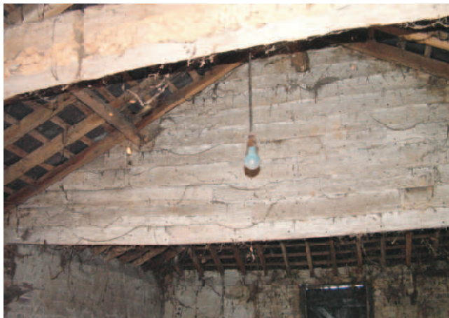
Timber and boarded infill above removed division wall.
