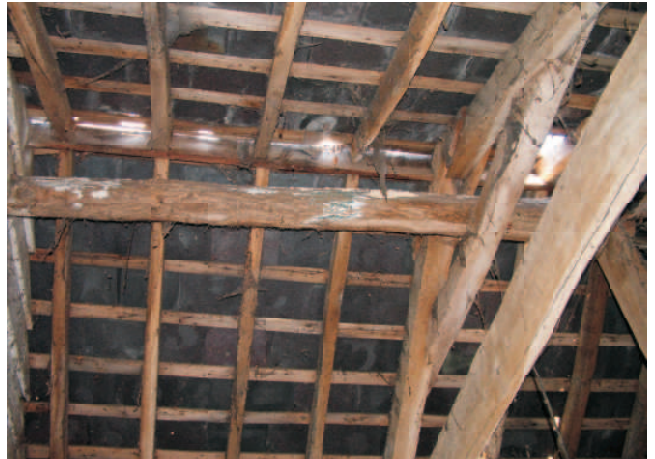
Good roof, simple trusses, slate covered.
