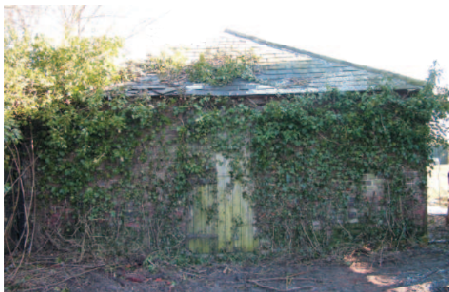
Western hipped end of building with door to Goose Yard.
