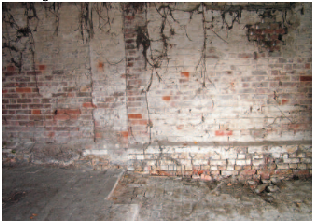
Brick floor at removed division wall.
