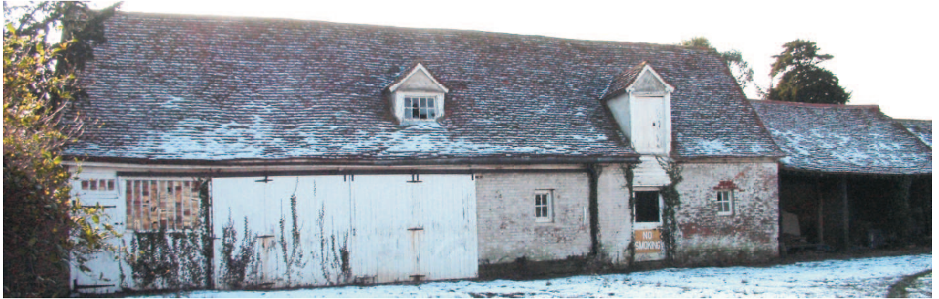
Building C to south. Carriage sheds with stable to right and Hay loft above. Dormer window to upper room.
