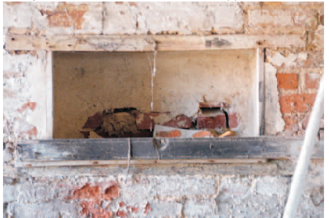
Wall niche in east wall - framed in timber & plastered.
