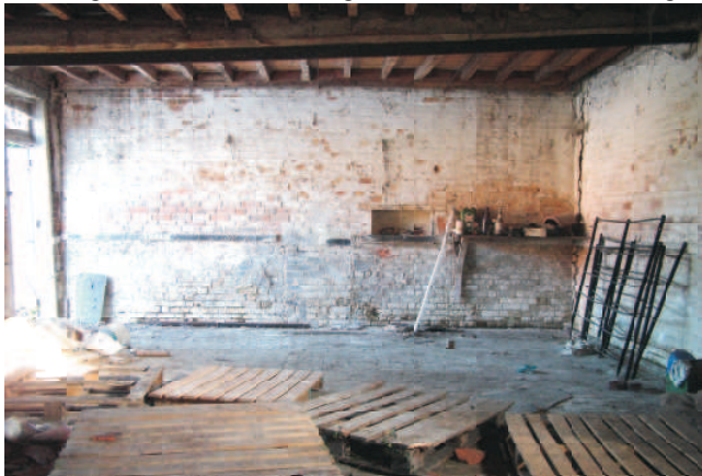
East wall of Carriage shed with infilled fireplace.
