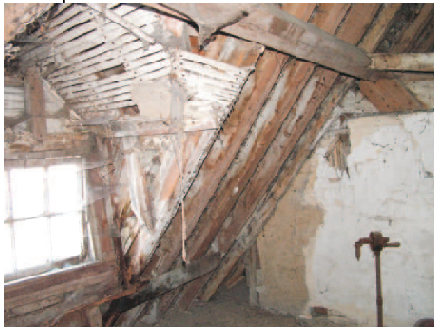
Dormer window to living room in north roof.
