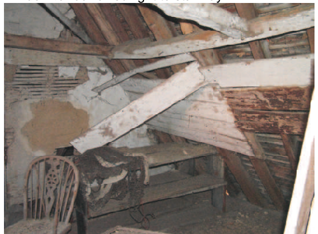
Boarded finish to south roof, plastered finish to east.
