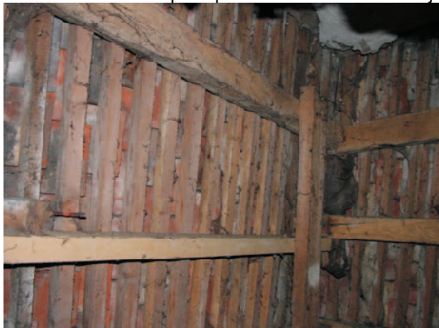
Roof at stair landing for lost stack.
