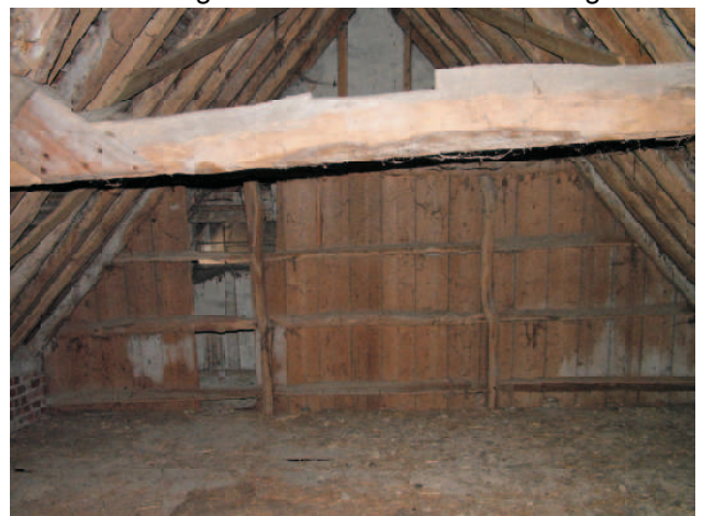
View to east boarded out from stair landing.
