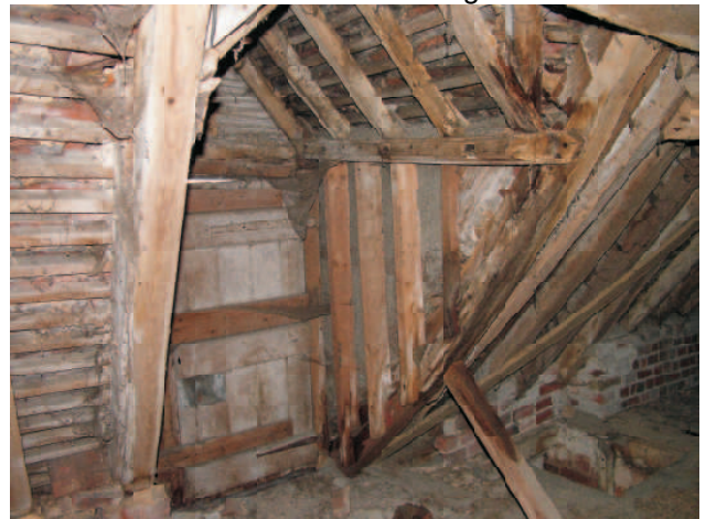
View to loading door with ladder access to right.
