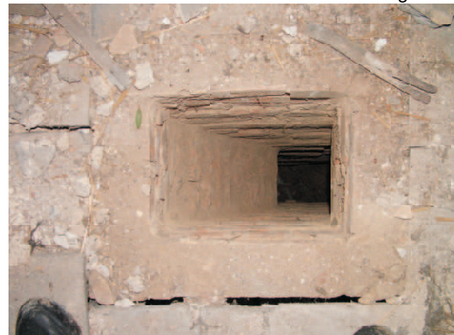
View down removed stack.
