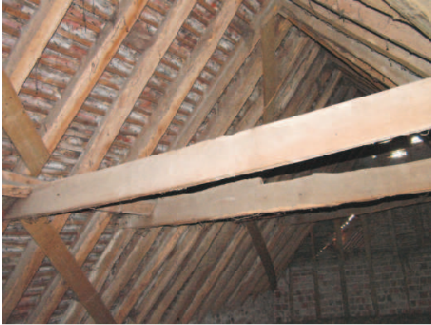
Building C. Hay loft over stables. Roof structure.
