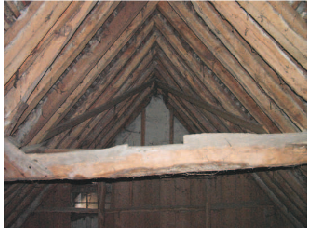
Roof above collars viewed to west gable.
