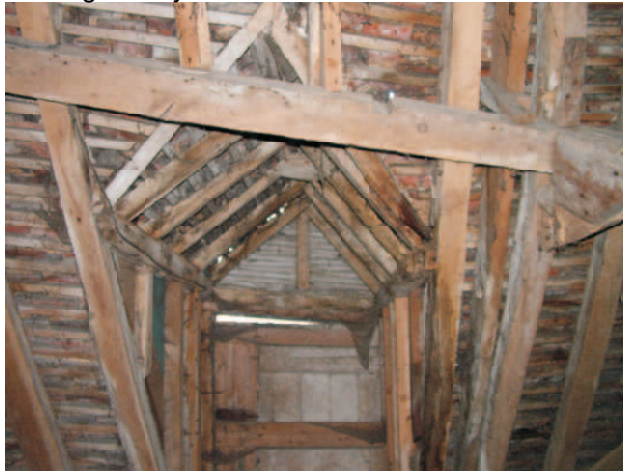
Dormered loading door possibly early C19 boards.
