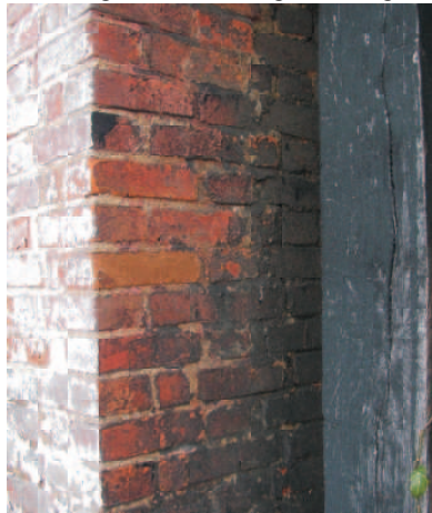
Front corner of wall east build.
