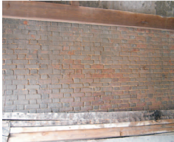
End wall of east build showing good Flemish bond brickwork & gable above.
