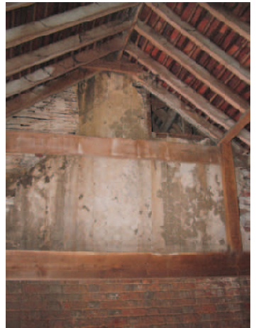
End wall of east build showing good Flemish bond brickwork & gable above.
