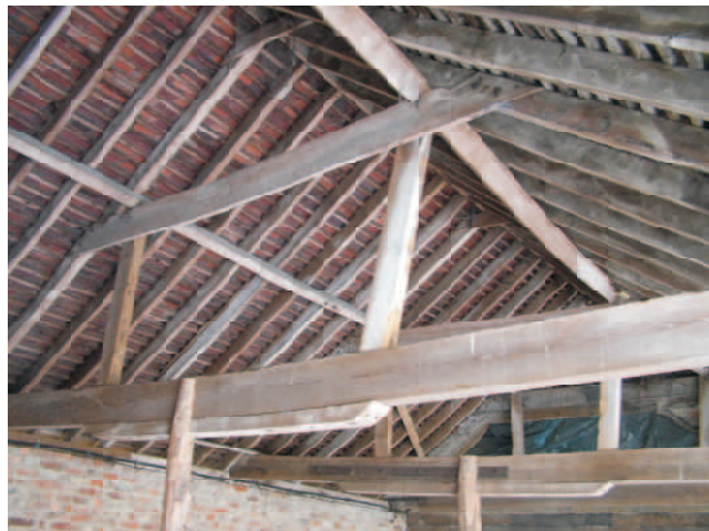
Good elm roof side purlin with collars & Queen struts.
