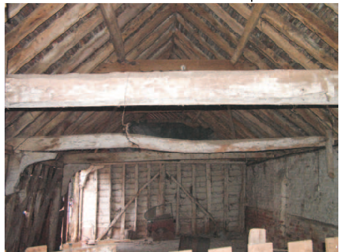
East wall timber framed much reused timber.
