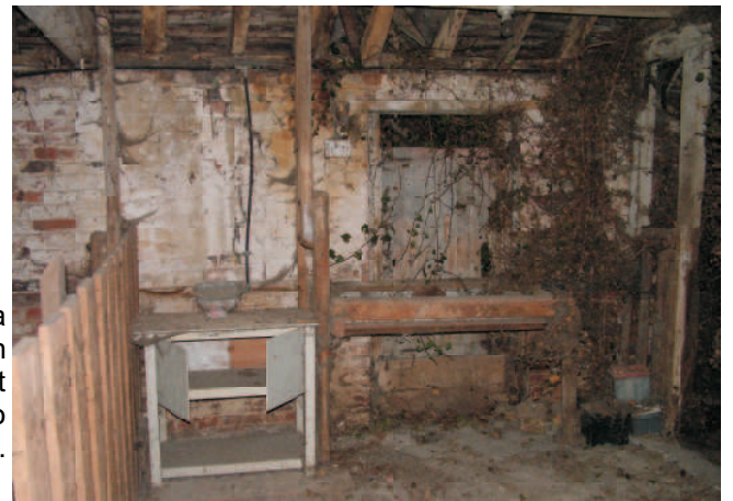
East wall timber framed much reused timber.
