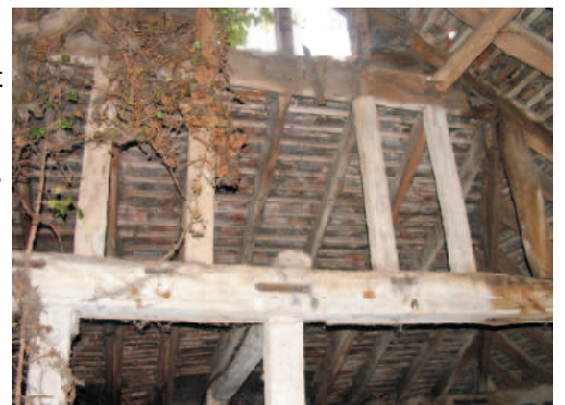
Added lean-to to the west end with stall divisions having linking gates for selection of animals or as calve pens. End wall of cowhouse opened up to allow access.
