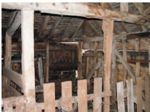
Added lean-to to the west end with stall divisions having linking gates for selection of animals or as calve pens. End wall of cowhouse opened up to allow access.
