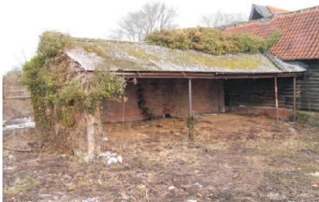
Open shed, The Pig Yard, attached to west wall of barn.
