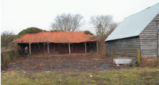
Western shelter shed with bricks remains and new build to east. Remnant of yard wall to west.
