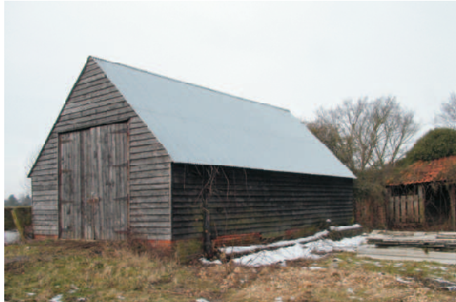
Modern build, timber framed and clad with corrugated iron roof. Some of the plinth bricks possibly from an earlier brick building with remains forming a brick walled yard area to the north between shelter sheds.
