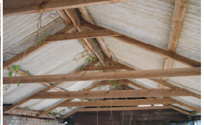
Simple modern roof for asbestos sheet covering.
